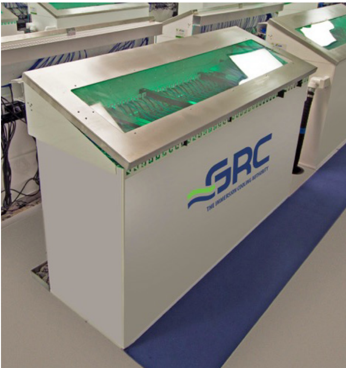
Fig. 3. The immersion cooling system at the Laboratory for Physical Sciences, like the one pictured above, uses mineral oil to cool IT equipment. (Photo used with permission from Green Revolution Cooling: grcooling.com.)
