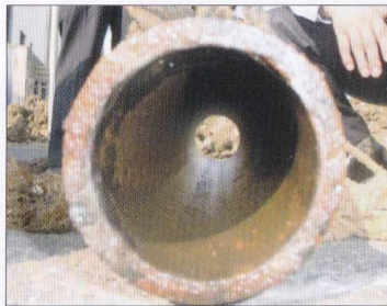
3 years after the installation (October 26, 2005)
