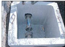
Installing Scale-Buster/ installing pipe annuli
